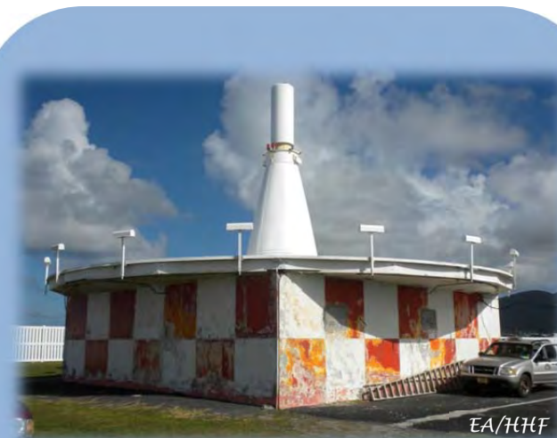
Figure 3.4 - The VHF Omni-directional Radio and Tactical Air Navigation system at the Pago Pago airport was disabled by the 2009 SPT impeding aerial navigation to Tutuila. (Photo: EA/HHF)
