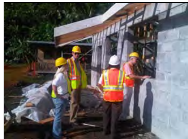
Figure 3.18 - One of the 41 FEMA-funded replacement homes under construction. The Federally funded reconstruction of new homes in American Samoa faced challenges with land use constraints. (Photo: FEMA, N.D.)
